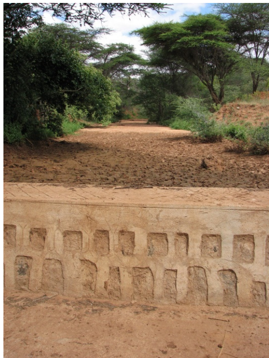
Fig. 3 A sand dam in Borana.
