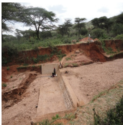
Fig. 4 A sand dam constructed under the ADAPTS project
